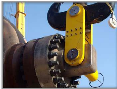
Static equipment Erection
