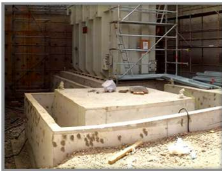
Foundation for Equipments
