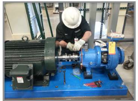
Rotary equipment Erection
